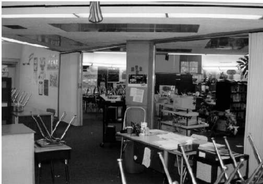
FIGURE 9. Open Plan Classrooms While advantageous for certain teaching methods or student interaction, they have serious drawbacks acoustically. Although partial-height partitions or operable partitions eliminate visual distractions, they provide very little noise reduction between classrooms.
